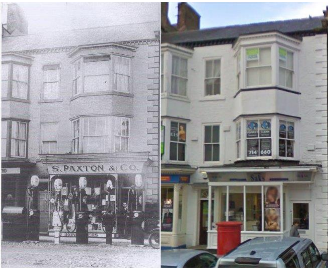
Figure 54 – Sep's Ironmongers and fuel pumps – in 1940s and in 2010.
