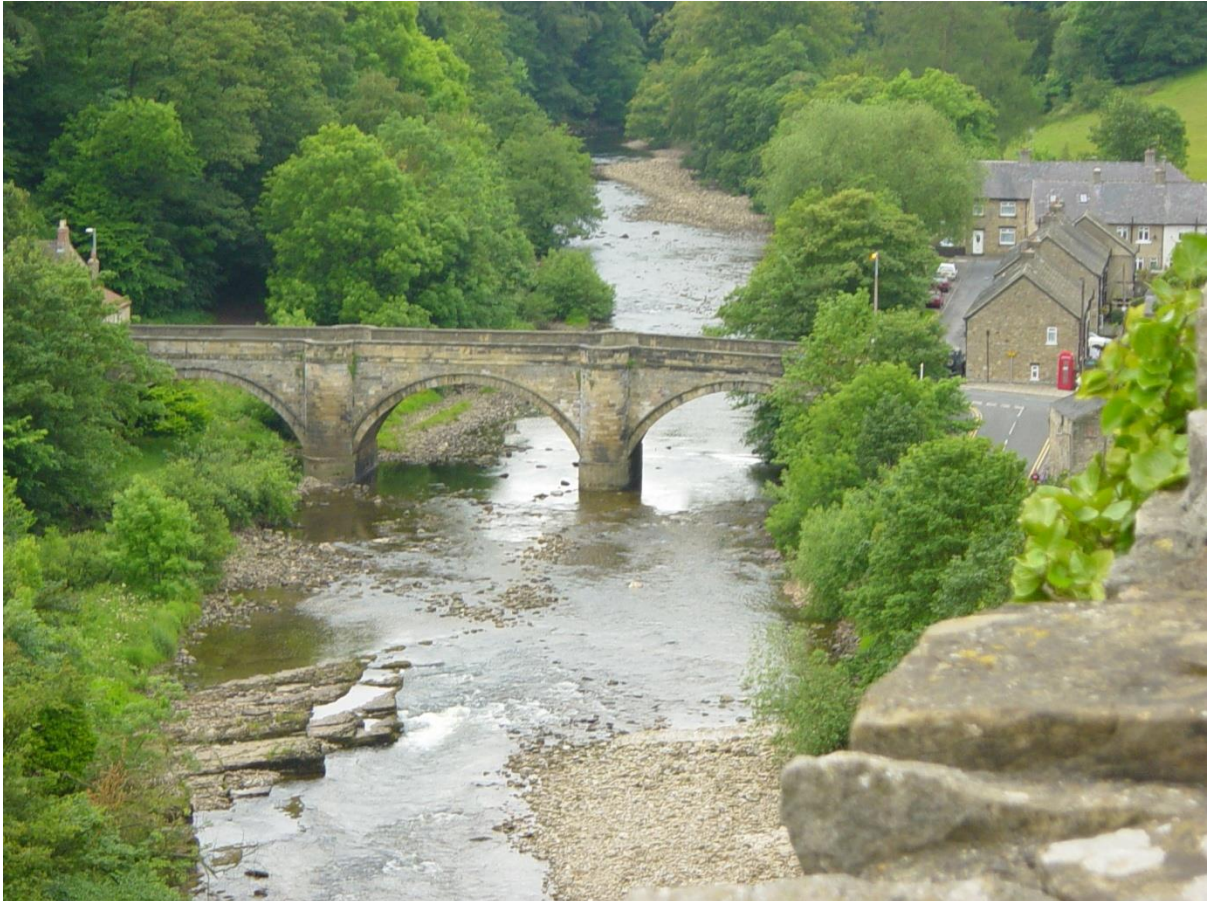
Figure 31 – The River Swale and Green Bridge from Castle Walk
