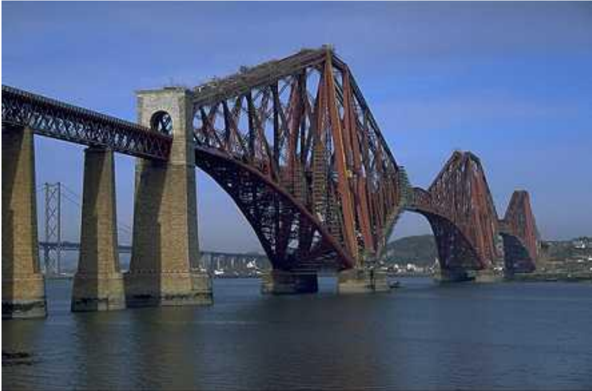
Figure 115 - The Forth Rail Bridge (Wikimedia Commons)
