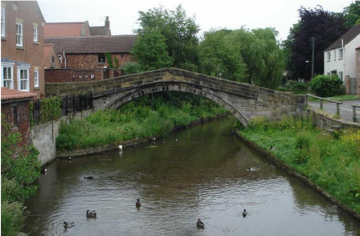
Figure 53 - Pack Horse Bridge over River Leven at Stokesley ( www.yorkshiremoors.co.uk )
