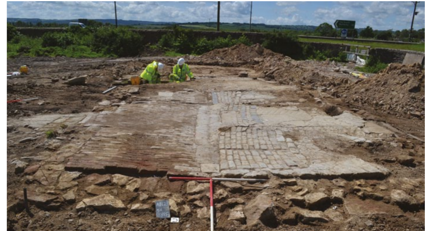
The former byre at Scurragh House during recording after demolition.
