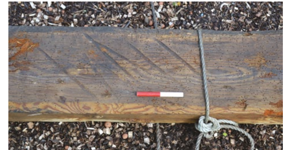
Marks of timbers removed during the demolition of Scurragh House. Such marks possibly resulting from the wood being imported from the Baltic.
